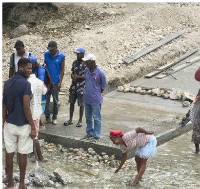
Road Construction: The main road into B-R crosses the "little river," a tributary of the river which is spanned by the pedestrian bridge. Unfinished pavement and an unstable river bed created a big problem for motorized and foot traffic. This year community leaders finished paving the road on both sides of the river than across the river bed, a feat of engineering savey.
