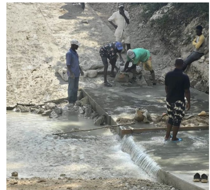
Road Construction: The main road into B-R crosses the "little river," a tributary of the river which is spanned by the pedestrian bridge. Unfinished pavement and an unstable river bed created a big problem for motorized and foot traffic. This year community leaders finished paving the road on both sides of the river than across the river bed, a feat of engineering savey.
